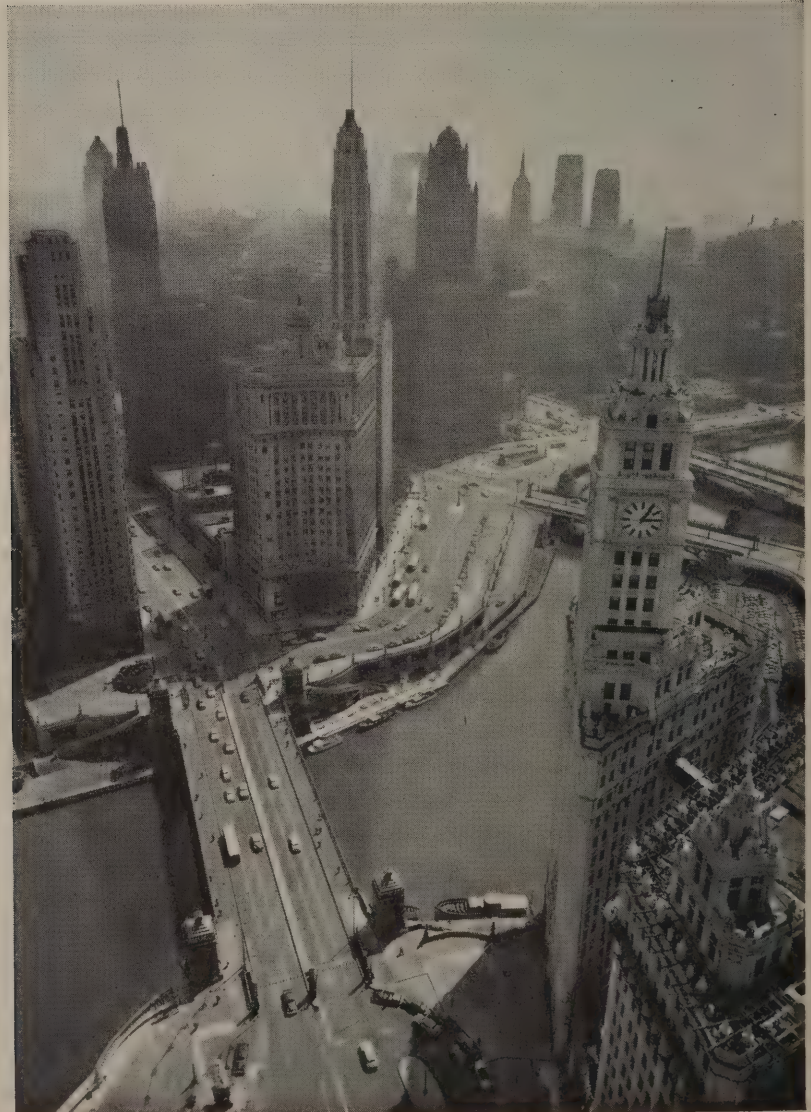
246 '... down town areas of such intrinsic power and character that they have retained their magnetism.' (Chicago. Bordering the far side of the river there is another wide highway underneath the road visible in the photograph).
